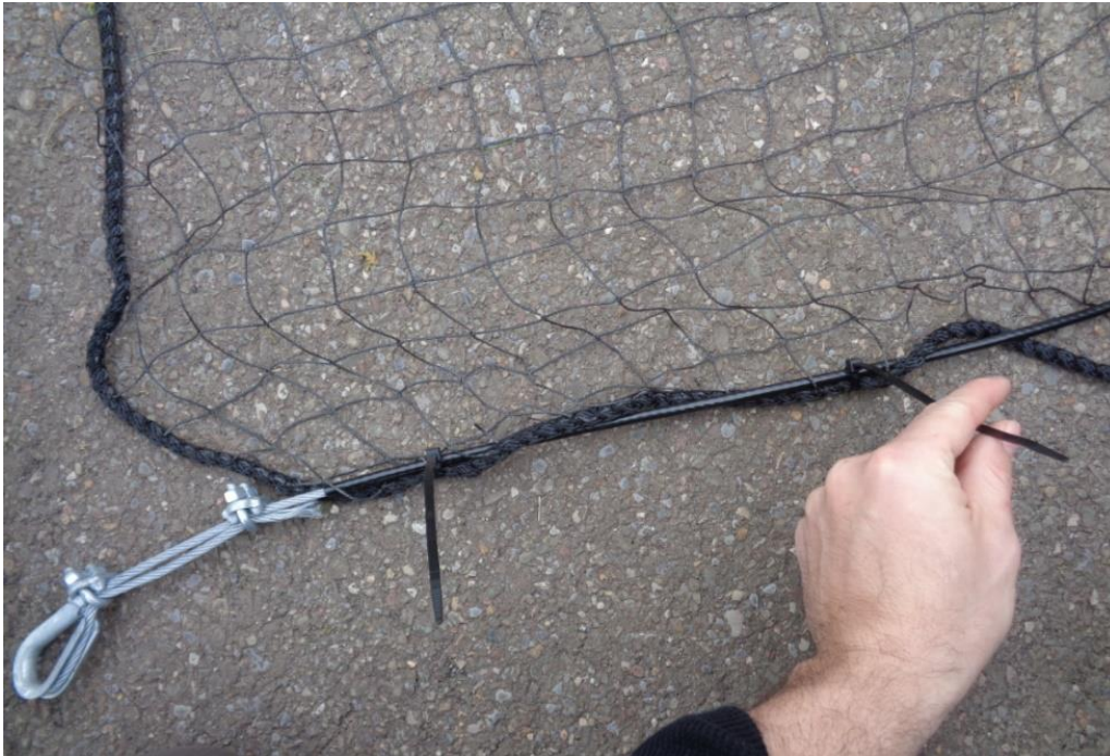
Figure 8 - Wire Rope to Bottom of Net Assembly
